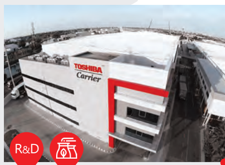
TCTC – ENGINEERING CENTRE
