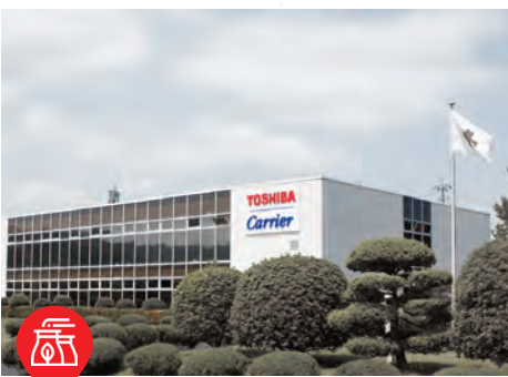
TCC – PRODUCTION FACILITIES
