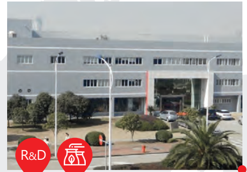
TCAC – PRODUCTION FACILITIES
